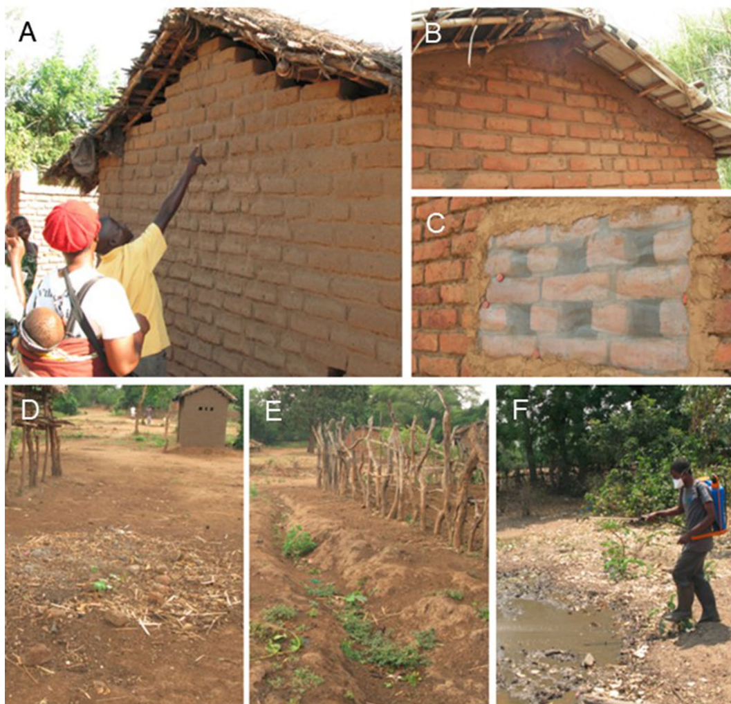
Fig. 2 House improvement (top panels) and larval source management (bottom panels). A Pre-intervention; B closed gable; C screened ‘windows’; D former water body filled with soil; E drainage passage created to prevent standing water; F trained LSM committee member applying Bacillus thuringiensis israelensis to water bodies. (Reprinted with permission from van den Berg et al. [28])
